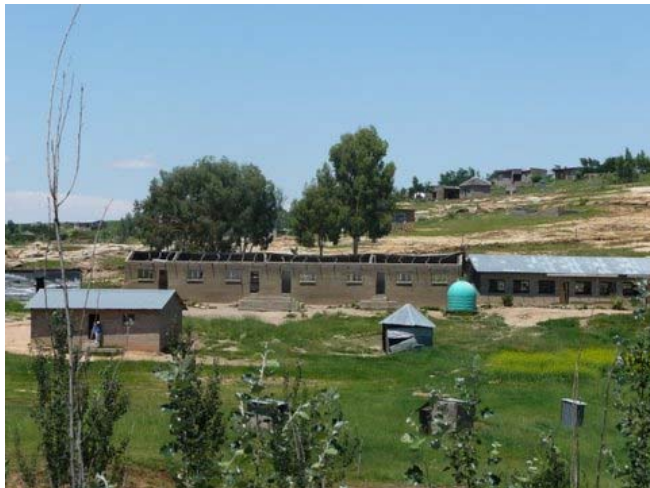
Motati School – roof destroyed by winter storms
